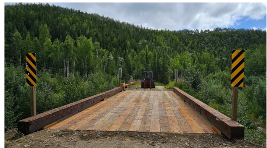
Heavy equipment section maintains the Cache Creek bridge in TVSF. Egil Fjellheim/DFFP
